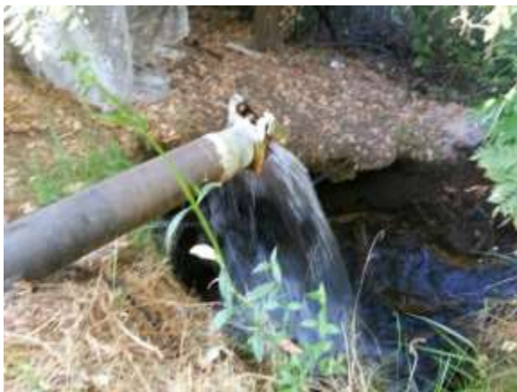
Figure 3: Outlet pipe into Bushy Lake from Cal Expo.
